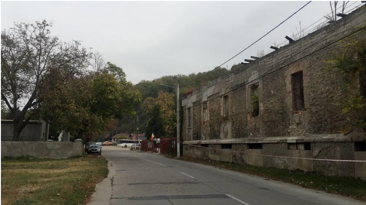
Fig. 7 Aspects of existing vegetation around the MFS building site
